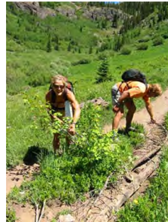
Patsy and Andy cutting brush and blocking a braided section of trail.
